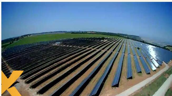
PV Carolinas (Guadalajara) 10 MWp
