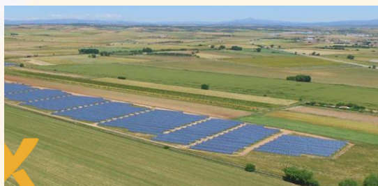
PV Cañamares (Guadalajara) 5 MWp
