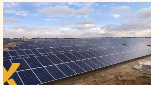
PV Carolinas (Guadalajara) 10 MWp
